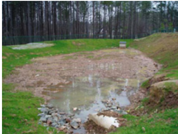
Figure 8. Existing dry ponds can be great retrofits (SR 1-3)
