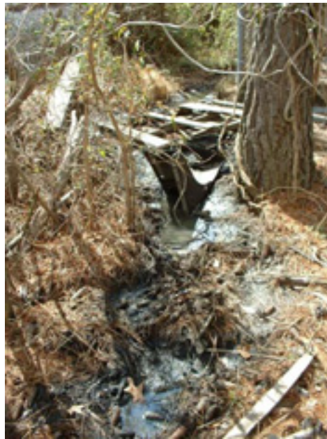
HS-4-2 Durham Area Transport Authority (DATA): Uncovered diesel fueling area lacked secondary containment. Diesel was observed leaking across the parking lot into the storm drain inlet behind the bldg.
