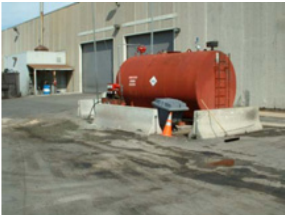
HS-1-2A and HS-2-2 At Park East Ventures (left) no pollutant source was confirmed, but rusty, uncovered fuel storage tanks and oil/antifreeze barrels were placed near a highly eroding area. At B & R Construction (right), unlabelled barrels contained unknown materials.
