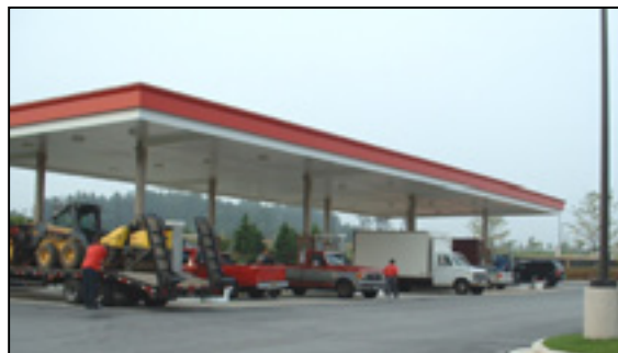
Figure 1: Covered Retail Gas Operation Without Containment for Potential Spills
