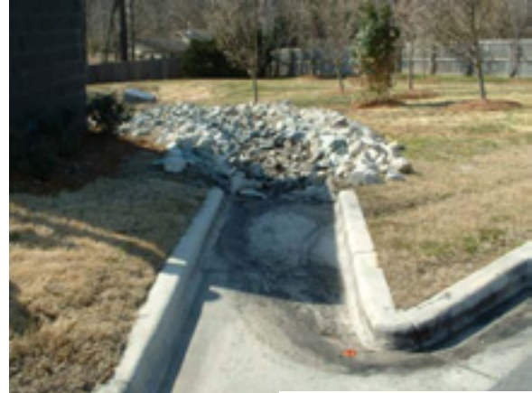
HS-3-1 Grease globules and wash water stain in channel and riprap leading to BMP at Cookout fast food restaurant. (above and left)
