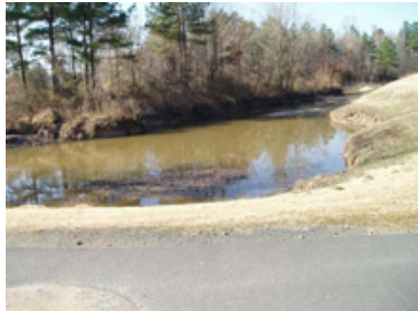
SR-5-9 involves enhancing existing golf course water features to provide water quality treatment for runoff from the adjacent subdivision.
