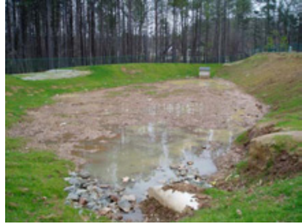
SR-1-3 Existing Dry pond at Pendleton Apartments.
