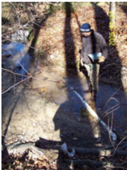
RCH2-10 Outfall of Failing Sand Filter
