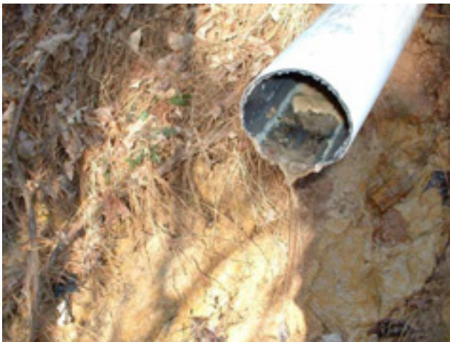
RCH2-10 Outfall of Failing Sand Filter
