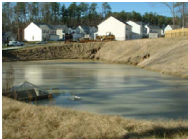
RCH2-12 Stormwater pond in use as sediment basin (right)
