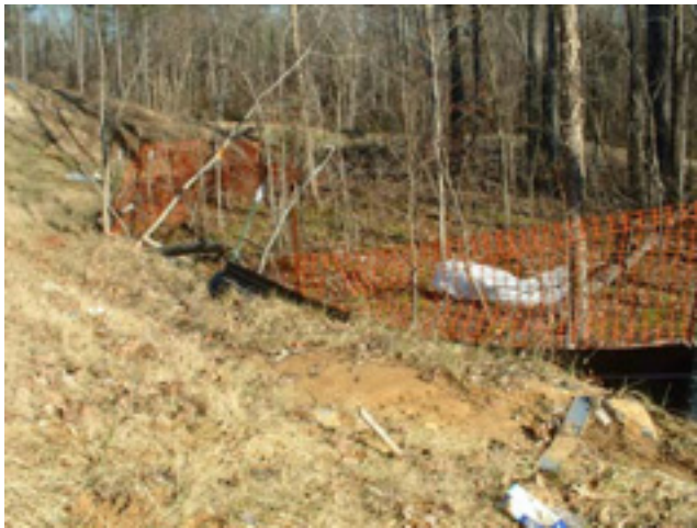
RCH2-12 Unmaintained erosion and sediment controls (left photo). Upstream area was graded and seeded, but has not yet stabilized. The sediment load carried down this hill overwhelmed the silt fence and is filling in the sediment basin (right photo).
