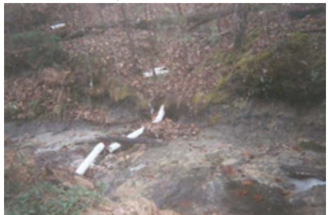
RCH5-8 PVC sanitary sewer laterals in stream (above and left)
