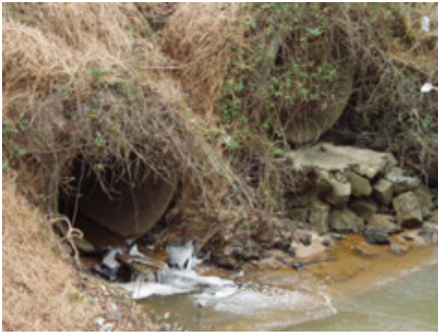
RCH3-4 Illicit discharge – wash water (left) RCH3-7 Illicit discharge - Paint dumped in stream (right)
