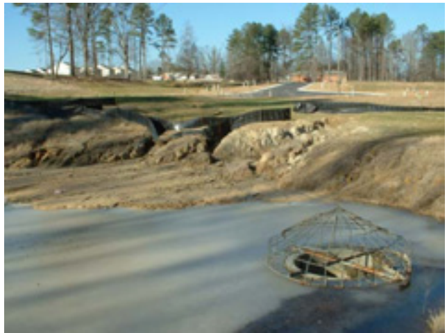
RCH2-12 Unmaintained erosion and sediment controls (left photo). Upstream area was graded and seeded, but has not yet stabilized. The sediment load carried down this hill overwhelmed the silt fence and is filling in the sediment basin (right photo).
