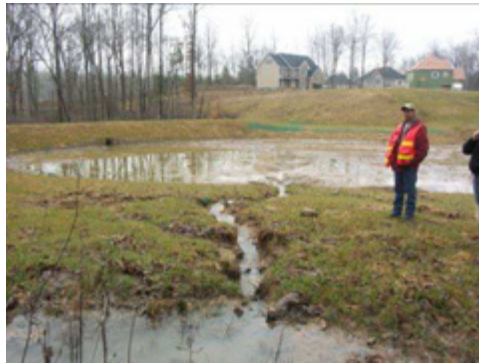
MI-301 (left) This approved in-stream pond at Brightleaf destroyed a natural stream and buffer. MI-303 (right) This pond in Brightleaf demonstrates the typical unimaginative site layout and short flow path. MI-303 is recommended for a retrofit to lengthen the flow path.
