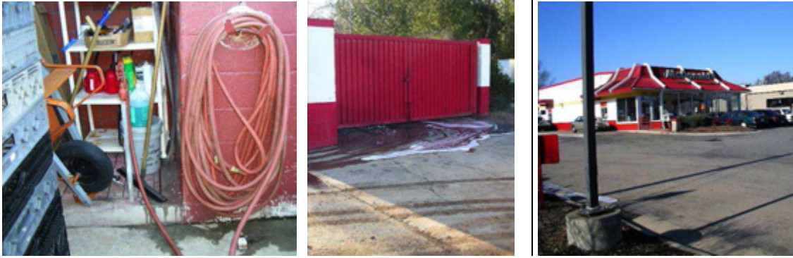
H-300 McDonald's at Route 70 and Mineral Springs Road. Dumpster area is set up for washing (left). Wash-water leaves the dumpster area (middle) and flows through parking lot to storm drain inlet near parking lot entrance from Route 70 (right).
