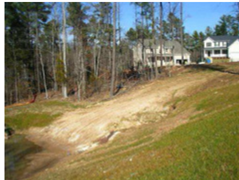
One of the 40 one-year detention ponds in Brightleaf. The small volume and short flow path (left) will make water quality retrofits difficult. The steep slopes (right) impede maintenance access.
