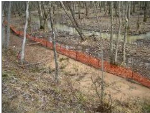
MI-309 (left) Silt fence at bottom of slope is adjacent to stream and wetland and filled to brim with sediment. OT-120 (right) Bulging silt fence at edge of Snappy's Lake.
