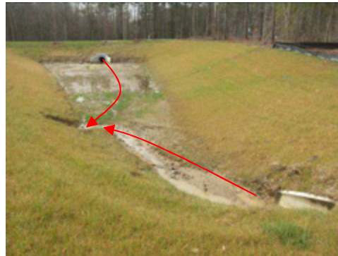
MI-301 (left) This approved in-stream pond at Brightleaf destroyed a natural stream and buffer. MI-303 (right) This pond in Brightleaf demonstrates the typical unimaginative site layout and short flow path. MI-303 is recommended for a retrofit to lengthen the flow path.
