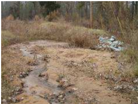
MI-205 (left) Filled sediment basin lacks functional storage. Near IB-110 (right) Un-maintained inlet protection.
