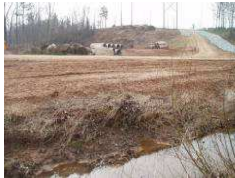
IB-210 Cleared buffer and road construction lacking S&E controls at Kingsmill Dairy.
