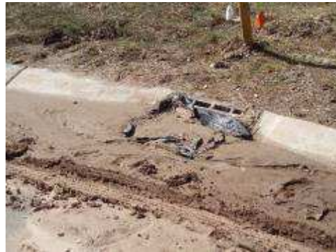
MI-205 (left) Filled sediment basin lacks functional storage. Near IB-110 (right) Un-maintained inlet protection.
