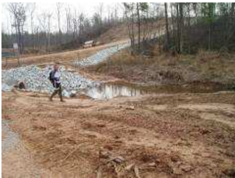
IB-210 Cleared buffer and road construction lacking S&E controls at Kingsmill Dairy.
