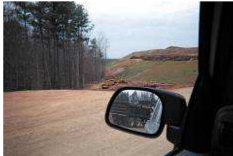
IB-210 Cleared buffer and road construction lacking S&E controls at Kingsmill Dairy.
