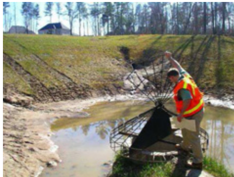
One of the 40 one-year detention ponds in Brightleaf. The small volume and short flow path (left) will make water quality retrofits difficult. The steep slopes (right) impede maintenance access.
