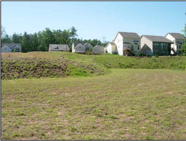
Figure 3. Land-clearing at IB-110.
